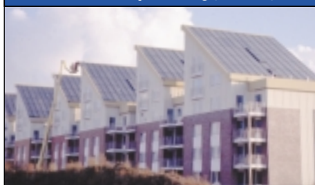
Fig 8: 1000 m 2 Solar Roof; North-south multi-family dwelling (Rostock)
