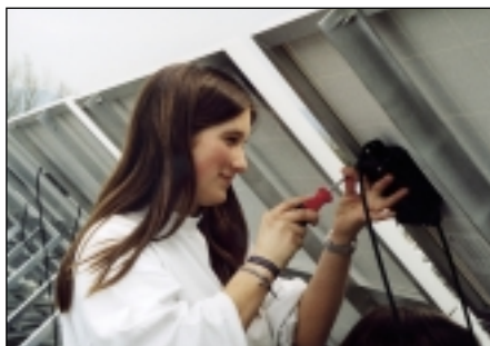
Fig. 10 Assembling a photovoltaic system at the Wentzinger Schulen
