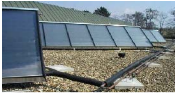
Solar thermal system under construction at a school
