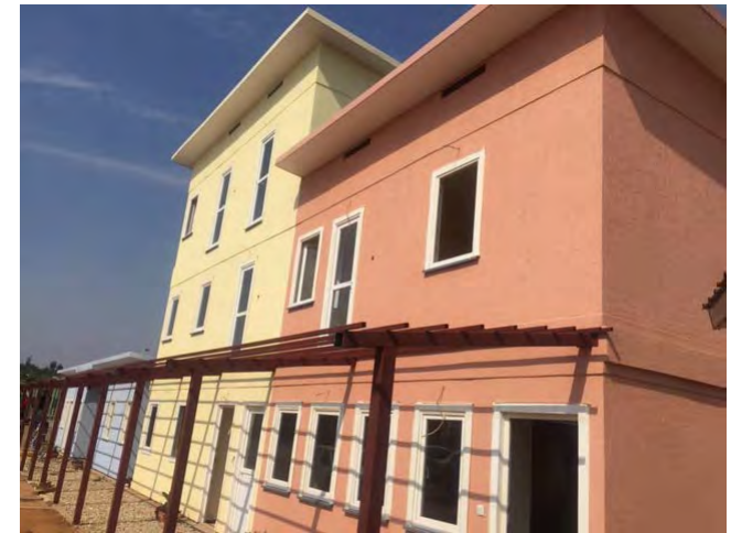
3 storey building in Kigali/Rwanda using STRAWTEC panels.
