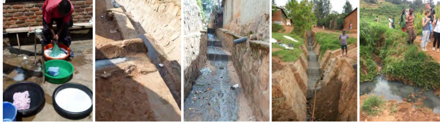
Problems of Greywater in Agatare
